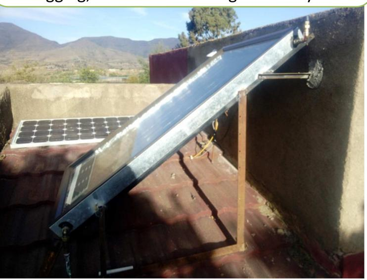
Due to lack of reticulated water, the low pressure pump system uses 50L cold-water storage tank on top to drive the hot water from the 50L geyser underneath
